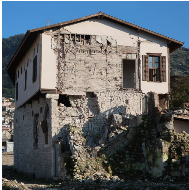
Rubble-stone masonry and Bağdadi exterior walls
