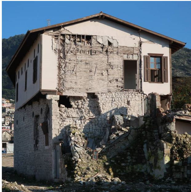
Rubble-stone masonry and Bağdadi exterior walls
