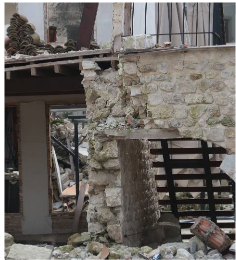
Rubble-stone masonry walls and wooden floors
