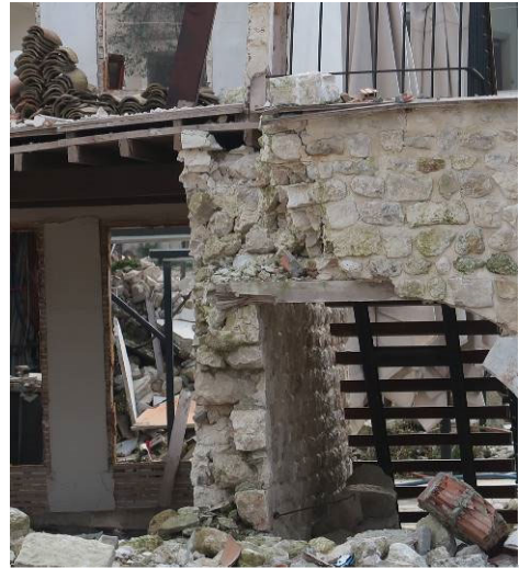
Rubble-stone masonry walls and wooden floors
